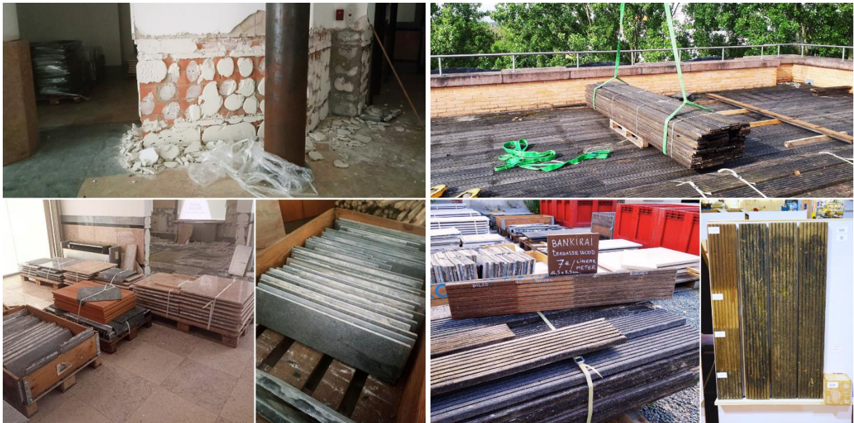
Twin Falls - Dismantling stone coverings © Rotor asbl
